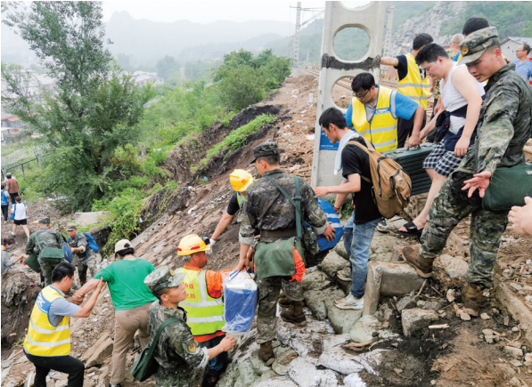
通号工程局集团成立应急救援抢险队、调派抢险车，开展丰沙铁路援抢险工作 CRSC Engineering Group has established an emergency rescue team and dispatched rescue vehicles to carry out rescue and repair work on the Fengtai-Shacheng Railway
